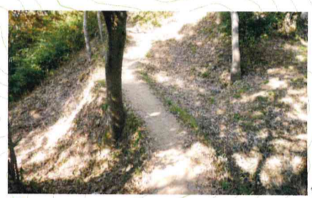
G Horikiri and Earthen Bridge Between Divisionland VIII lay double moats. The northern one has a narrow and winding earthen bridge.
