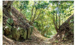
A long and wide Horikiri (steep moat) cut mountain ridge between Division VI and V for defending the northern area.
