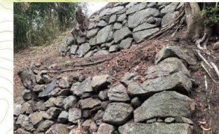
Two stepped stone walls supporting the eastern slope of Division III. This construction method would be effective to disguise two as one high wall seen from the bottom.
